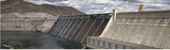
Electric Power Generation
